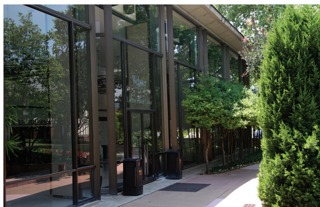
Exterior of the Loretto-Hilton Center, The Rep's primary performing venue.
